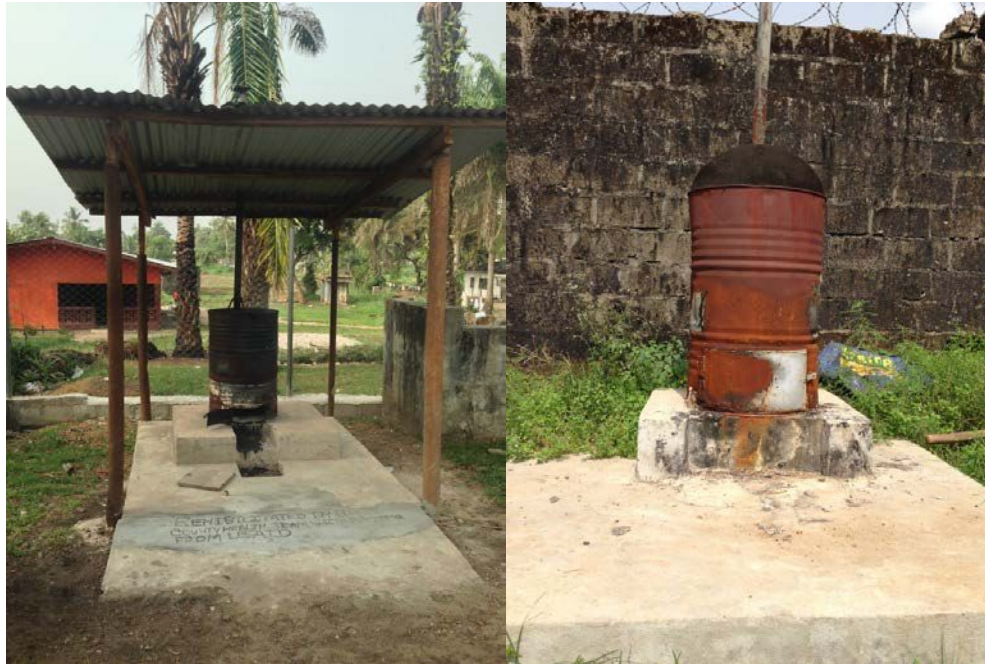
The incinerator at left (Incinerator 3) is oxidized and was expected to cease operating by September 2016. The incinerator at right (Incinerator 4) is no longer operational, and the facility was burning waste beside it, close to the clinic entrance. Photos: OIG (January 27 and 28, 2016)
